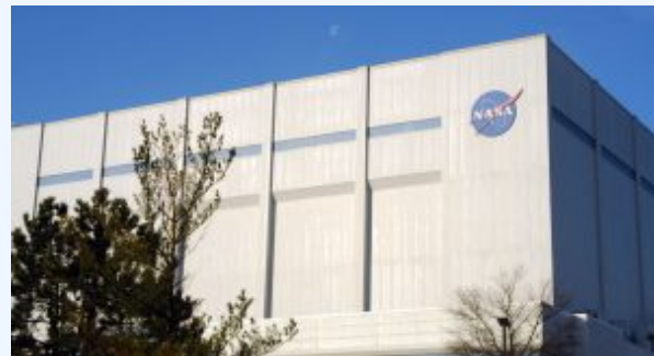
“Building 29 at Goddard Space Flight Center” by NASA Goddard Space Flight Centre is licensed under CC BY 2.0
