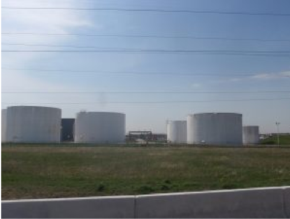
Figure 9.7: You might not know where the tiny town of Cushing, Oklahoma, is. But oil producers and traders around the world do. Cushing is one of the largest oil storage areas in the United States. Storage tanks like these cover more than nine square miles on the outskirts of the town (Davis, 2009). “ More Oil Storage ” by Anthony Easton , CC BY 2.0 .
