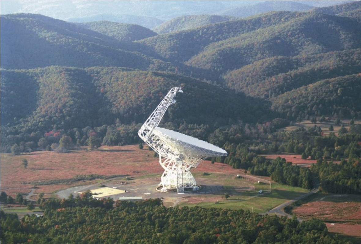
Figure 4.22. This fully steerable radio telescope in West Virginia went into operation in August 2000. Its dish is about 100 metres across.
