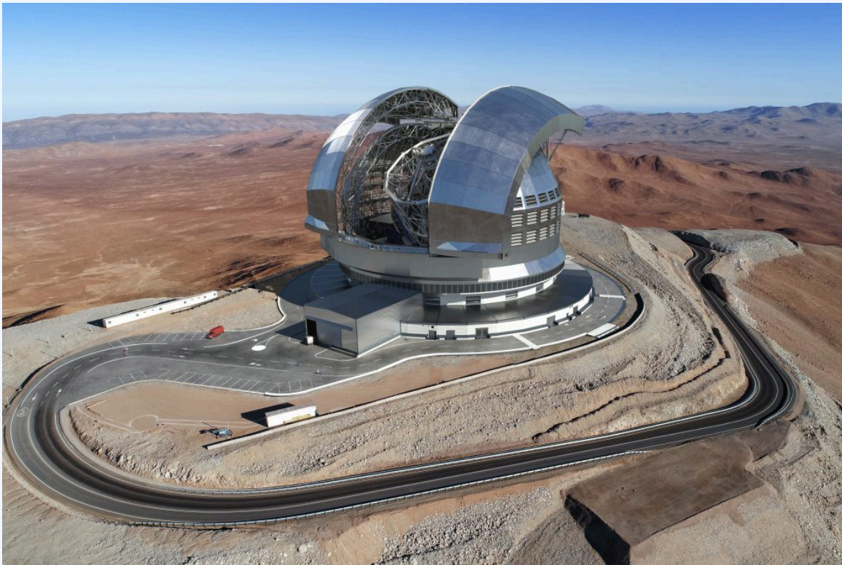
Figure 4.31. The primary mirror in The Extremely Large Telescope (ELT) is 39.3 metres across. The telescope is under construction in the Atacama Desert in Northern Chile. How the ELT will look like at Cerro Armazones by ESO , CC BY 4.0.
