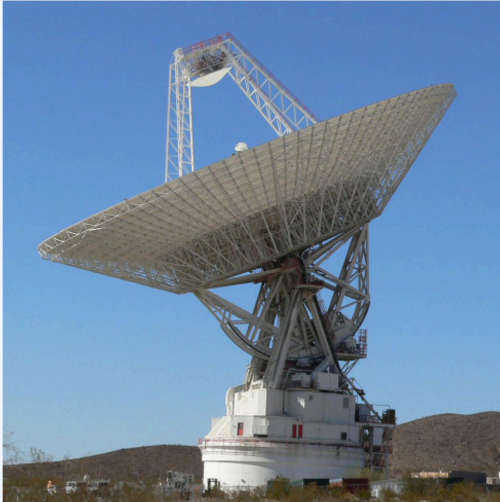
Figure 9.2. This dish-shaped antenna, part of the NASA Deep Space Network in California's Mojave Desert, is 70 metres wide. Nicknamed the "Mars antenna," this radar telescope can send and receive radar waves, and thus measure the distances to planets, satellites, and asteroids. Image by NASA/JPL-Caltech , NASA Media License .
