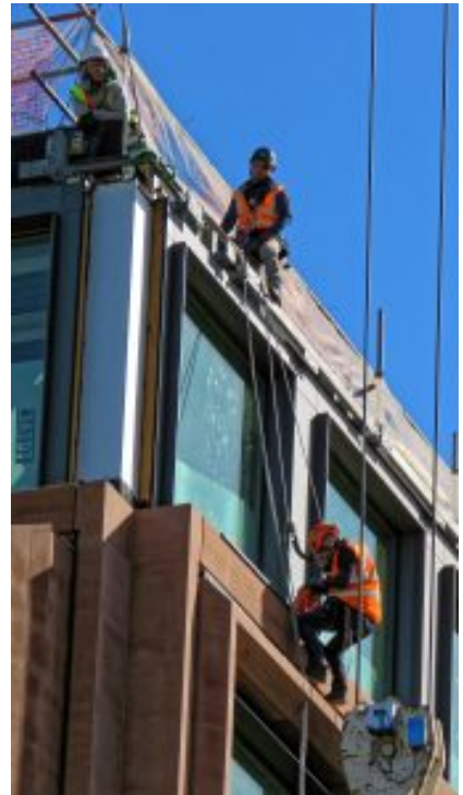
"Construction workers" by Acabashi, CC BY-SA 4.0
