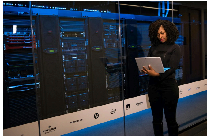
Big Data Processing (server racks)
