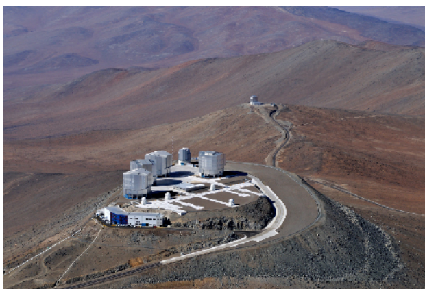
Figure 6.12. High and Dry Site. Cerro Paranal, a mountain summit 2.7 kilometers above sea level in Chile's Atacama Desert, is the site of the European Southern Observatory's Very Large Telescope. This photograph shows the four 8-meter telescope buildings on the site and vividly illustrates that astronomers prefer high, dry sites for their instruments. The 4.1-meter Visible and Infrared Survey Telescope for Astronomy (VISTA) can be seen in the distance on the next mountain peak. (credit: ESO)
