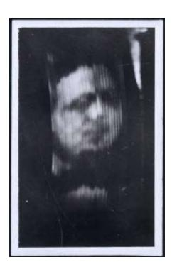
The low image resolution of John Logie Baird's mechanical television was a major disadvantage that led to the technology's replacement by electronic television systems.
