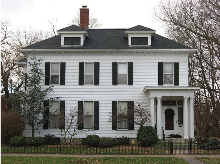
Historic Moss-Foster house, Colonial Revival style home in Sandusky, Ohio
