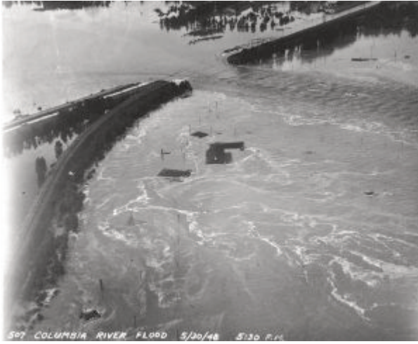
Water from the river flows into the city.
