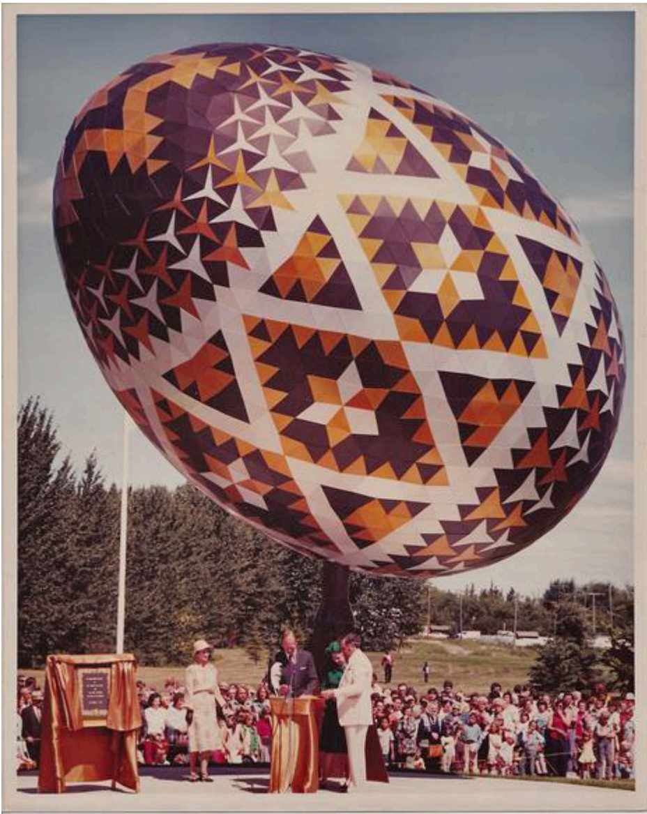
Vegreville Pysanka, constructed of 2D aluminum tiles – Geometry solved by Ron Resch and Robert McDermott
