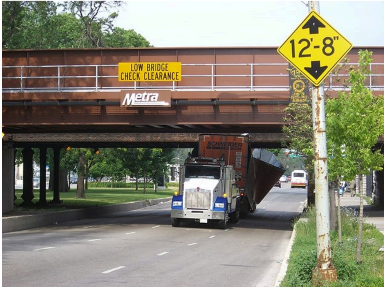
Transport Truck Trapped Under Low Bridge
