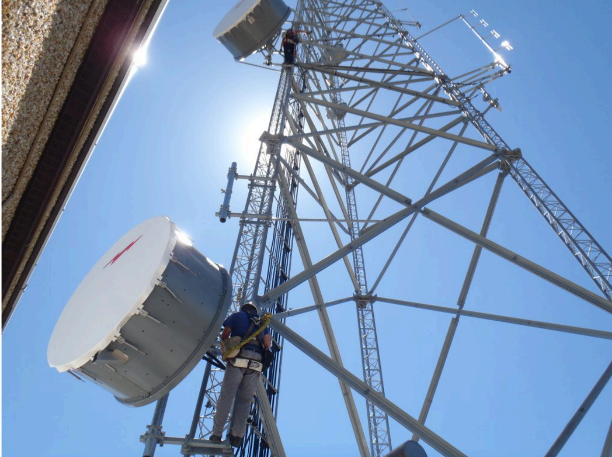
“Gogatha tower repair” by Oregon Department of Transportation , CC BY 2.0
