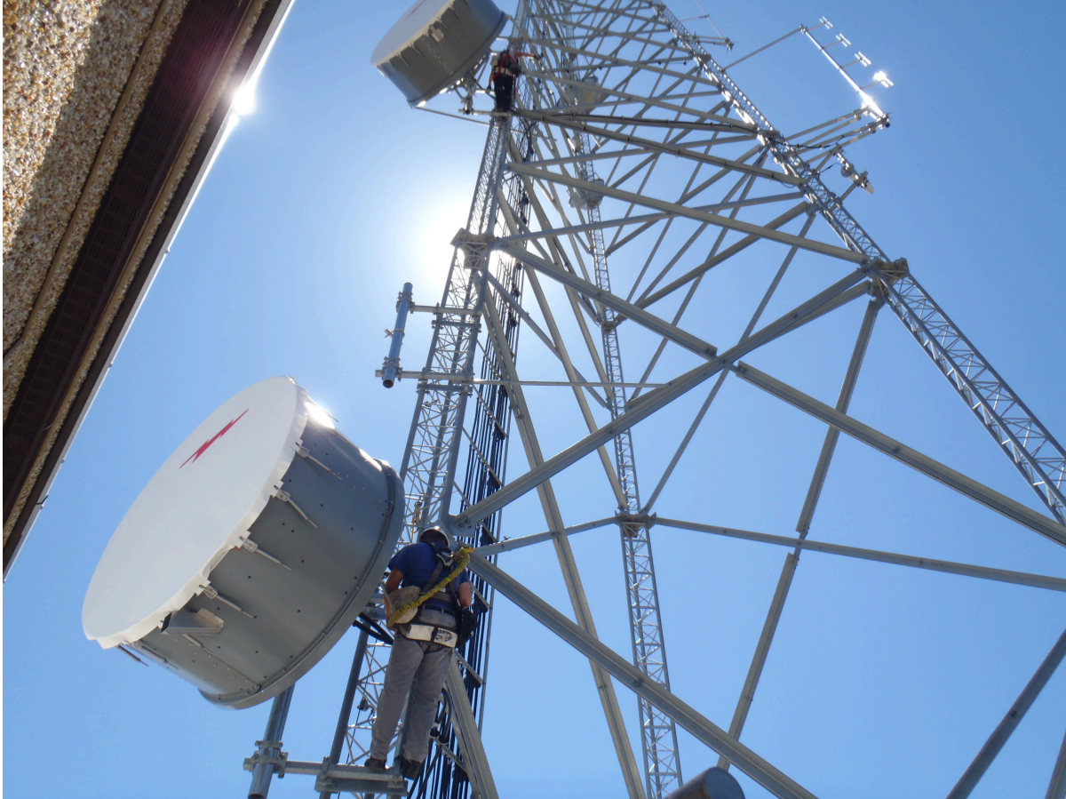
“Cogatha tower repair” by Oregon Department of Transportation, CC BY 2.0
