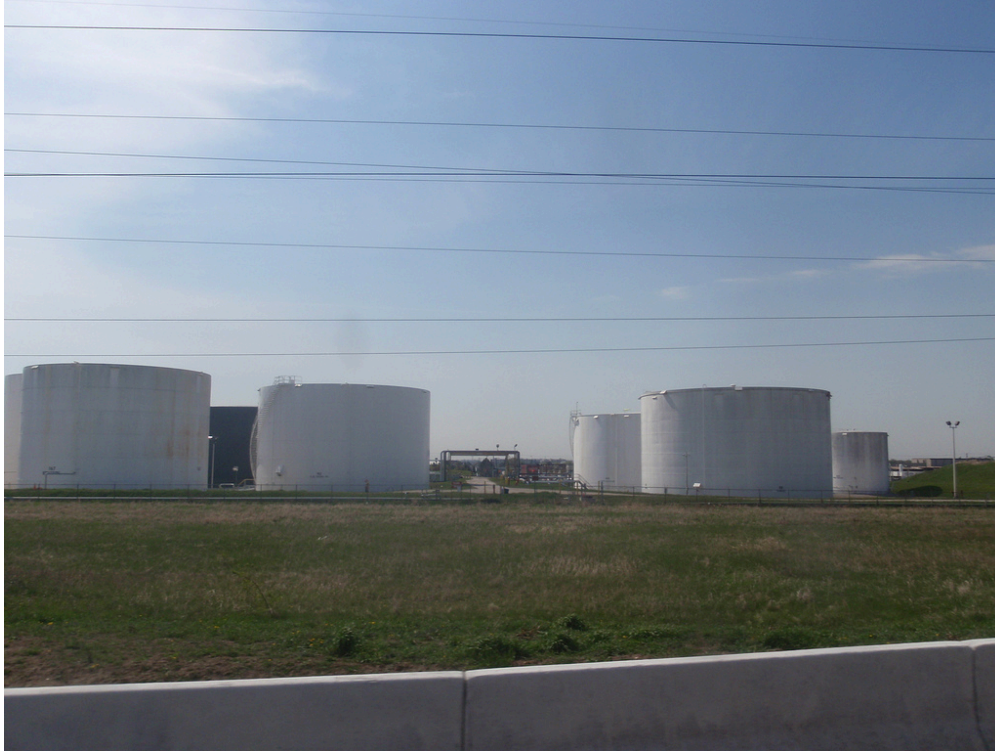
Figure 9.7: You might not know where the tiny town of Cushing, Oklahoma, is. But oil producers and traders around the world do. Cushing is one of the largest oil storage areas in the United States. Storage tanks like these cover more than nine square miles on the outskirts of the town (Davis, 2009). “More Oil Storage” by Anthony Easton, CC BY 2.0.
