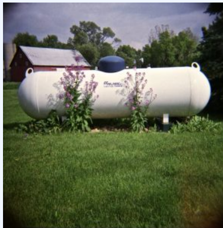
Figure 8.2a Propane is a fuel used to provide heat for some homes. Propane is stored in large tanks like that shown here. (credit: work by vistavision , CC BY-NC-ND 2.0 )
