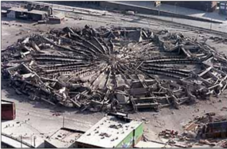
Fig. 5. Seattle Kingdome, Seattle, WA, after implosion.[35]
