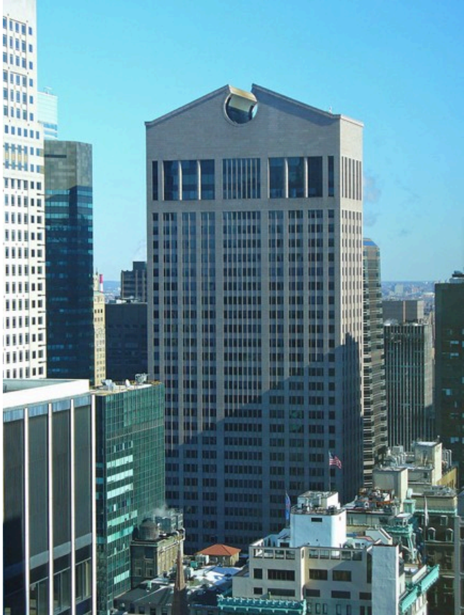
Philip Johnson, 550 Madison Avenue (formerly the AT&T Building), New York, 1982, Photo by David Shankbone, taken Feb. 19, 2007. CC BY-SH 3.0
