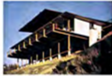
Here's how a house was built at Marin Bay, San Rafael, California. Steel for strength and permanence. This house can shrug off an earthquake, and didn't shudder when a helicopter landed on the roof.
