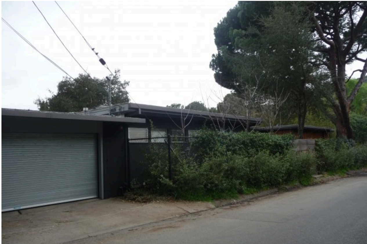
Walter Gropius and The General Panel Corporation, The General Panel Residence on North Nichols Canyon Road in the Hollywood Hills, 1951 https://www.laconservancy.org/locations/general-panel-residence
