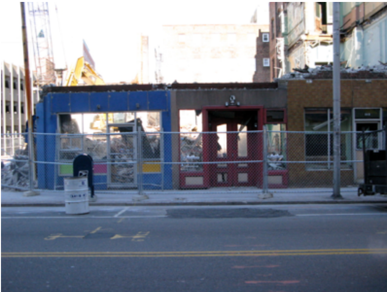
Fig. 6. All pictures, demolition of Talk of the Town, 2008. (Gabriela Salazar)
