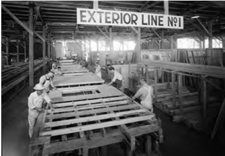
Figure 7 Kaiser Community Homes in Los Angeles, assembly line, c. 1946.
