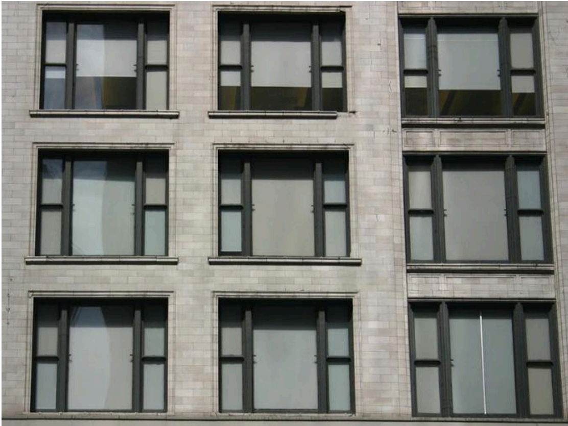
Chicago School window grid: The Chicago window combined the functions of light-gathering and natural ventilation; a single central pane was usually fixed, while the two surrounding panes were operable. Photo by J. Crocker, taken March 30, 2006. CC BY
