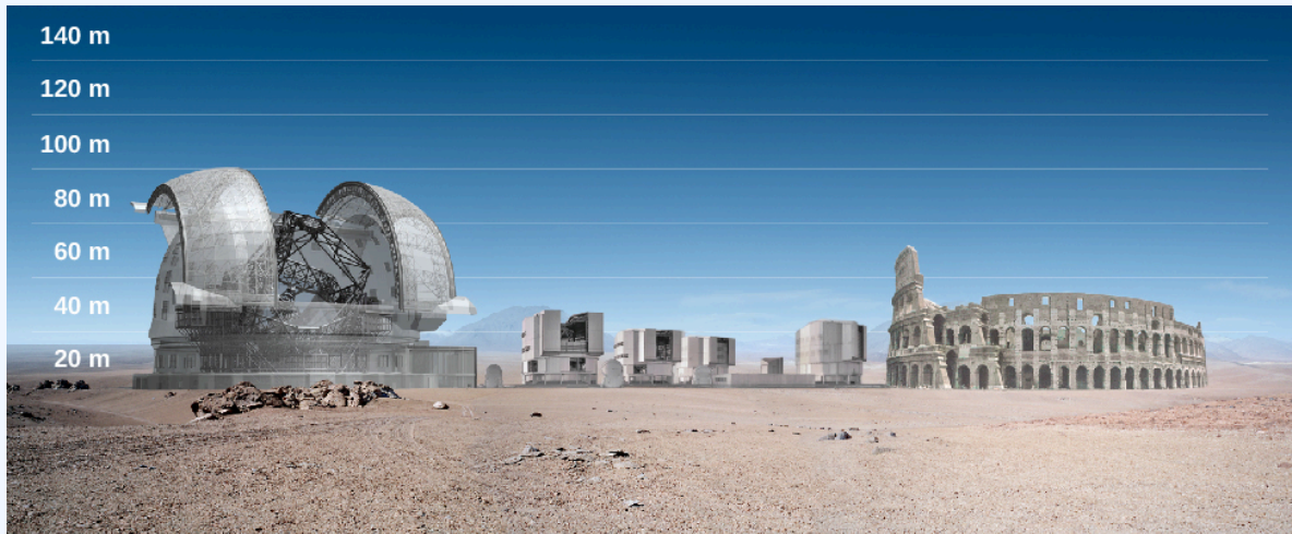
Figure 15.10. The European Extremely Large Telescope (E-ELT) is currently under construction in Chile. This image compares the size of the E-ELT (left) with the four 8-meter telescopes of the European Very Large Telescope (centre) and with the Colosseum in Rome (right). The mirror of the E-ELT will be 39 metres in diameter. Astronomers are building a new generation of giant telescopes in order to observe very distant galaxies and understand what they were like when they were newly formed and the universe was young. (credit: modification of work by ESO)
