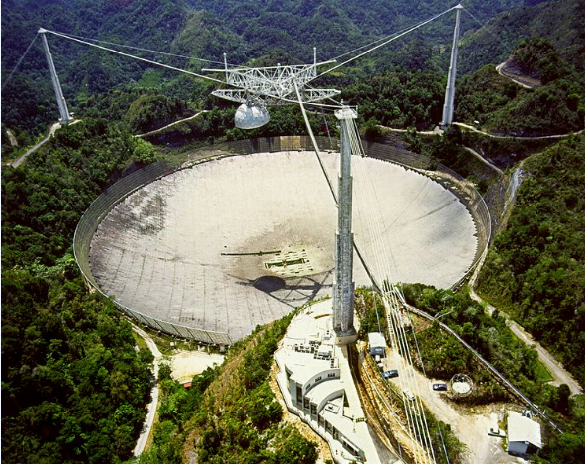
Figure 4.25. The Arecibo Observatory, with its 1000-foot radio dish-filling valley in Puerto Rico, is part of the National Astronomy and Ionosphere Center, operated by SRI International, USRA, and UMET under a cooperative agreement with the National Science Foundation. NASA Universe Arecibo Observatory Aerial View by H. Schweiker/WIYN and NOAO/AURA/NSF, CC BY 2.0.
