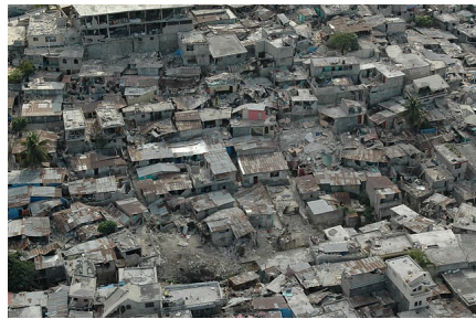
Haiti: Earthquake 2010, EU civil protection and humanitarian aid.
