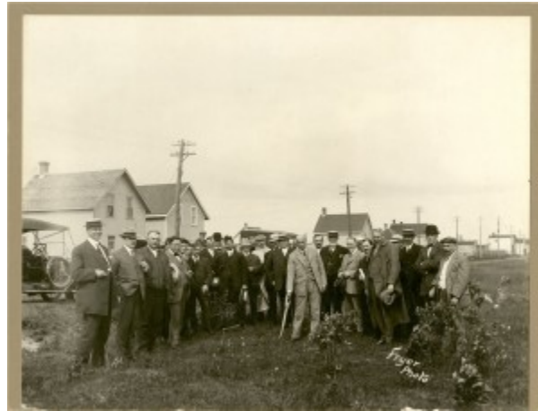
Figure 3.10 A sod turning in Thunder Bay in 1912 for a new Canadian Car and Foundry shop. Labour is not represented among the dignitaries.
