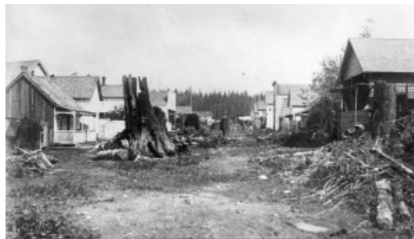
Figure 2.17 Fire trap. Hot weather, woodframe buildings, and an obvious abundance of tinder spelled disaster for Gastown/Granville/Vancouver in 1886.
