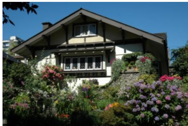
Figure 10.6 Hirshfield House in Vancouver's West End is an example of the Arts and Crafts style that recalled English village life rather than embracing modern city life.
