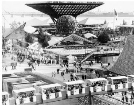
Figure 9.43 Expo '67 pavilions, built on specially created islands in the St. Lawrence.
