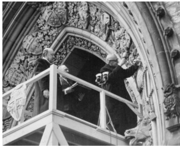
Figure 9.8 Prime Minister St. Laurent begins the process of carving Newfoundland’s coat of arms into the arch of the Parliament Buildings in Ottawa.
