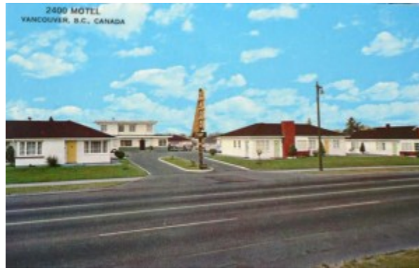
Figure 10.45 Motor hotels (motels) were part of the commercial infrastructure of the new tourism and car culture. Built in 1946 in south Vancouver, 2400 Motel is a distinctive, bungalow-style structure that was built, like other motels across North America, along a major corridor.
