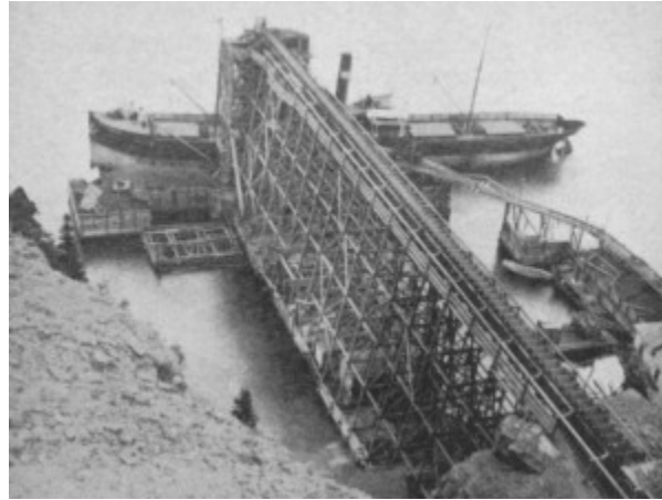
Figure 3.3 Iron ore from Bell Island is loaded onto a metal-hulled ship, ca. 1903.
