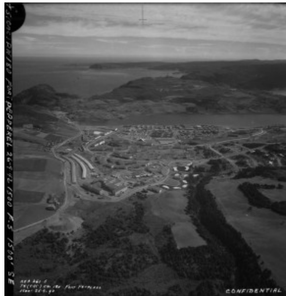
Figure 9.6 Building the massive American Fort Pepperell provided jobs to hundreds of Newfoundlanders and confirmed a United States presence in the former Dominion that drew it into the orbit of Washington.
