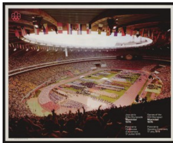
Figure 9.47 Opening ceremonies at the 1976 Olympics in Montreal, marred by extensive boycotts (in the end, only 92 nations participated). Construction cranes can be seen looming over the unfinished trunk of the stadium’s tower.
