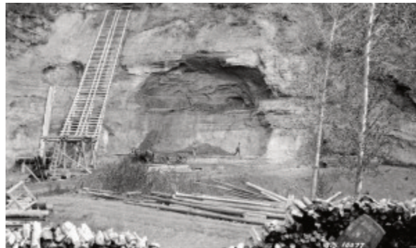
Figure 8.11 Oil sands were first exploited as a ready-made source of asphalt. Mining “tar sands” near Waterways, AB, in 1925.
