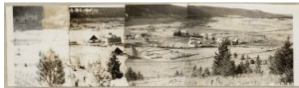
Figure 11.13 St. Joseph’s (Cariboo) Indian Residential School was established in 1891 as one of the several schools run by the Catholic Church in BC.
