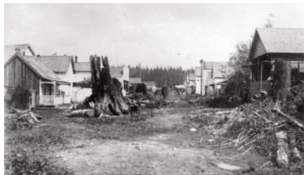
Figure 2.17 Fire trap. Hot weather, woodframe buildings, and an obvious abundance of tinder spelled disaster for Gastown/Granville/Vancouver in 1886.
