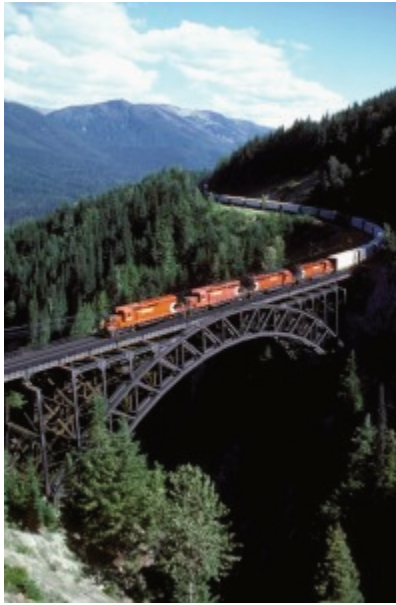
Figure 3.9 In 1893 the Stoney Creek steel bridge replaced a wooden trestle. It is a testament to the rising influence of engineering and improved materials in the late Victorian era. It is, as well, a graceful structure.
