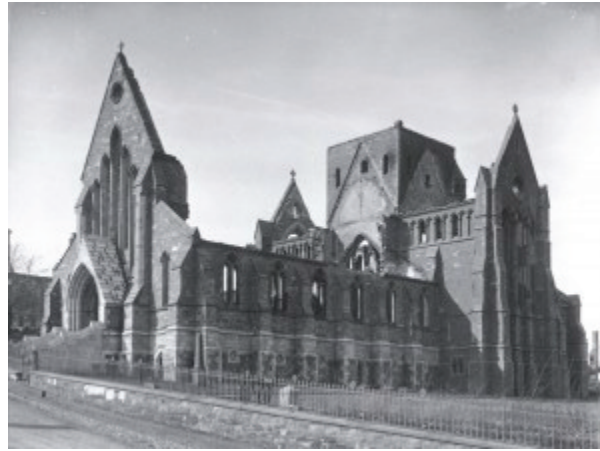
Figure 2.23 The shell of St. John's Anglican Cathedral after the 1892 fire.
