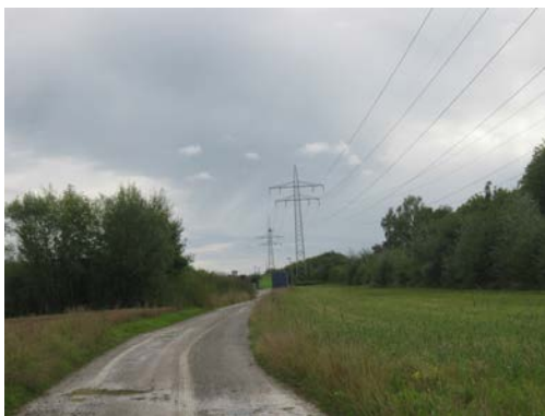
Figure 24.10 This high-voltage traction power line running to Eutingen Railway Substation in Germany radiates electromagnetic waves with very long wavelengths. (credit: Zonk43, Wikimedia Commons)
