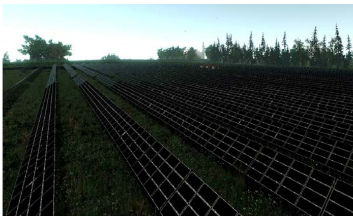
Figure 7.31 Solar cell arrays at a power plant in Steindorf, Germany (credit: Michael Betke, Flickr)
