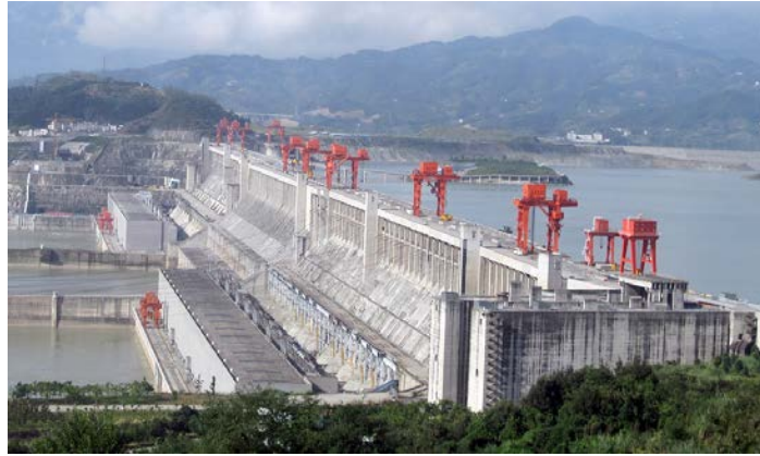
Figure 11.5 Three Gorges Dam in central China. When completed in 2008, this became the world's largest hydroelectric plant, generating power equivalent to that generated by 22 average-sized nuclear power plants. The concrete dam is 181 m high and 2.3 km across. The reservoir made by this dam is 660 km long. Over 1 million people were displaced by the creation of the reservoir. (credit: Le Grand Portage)
