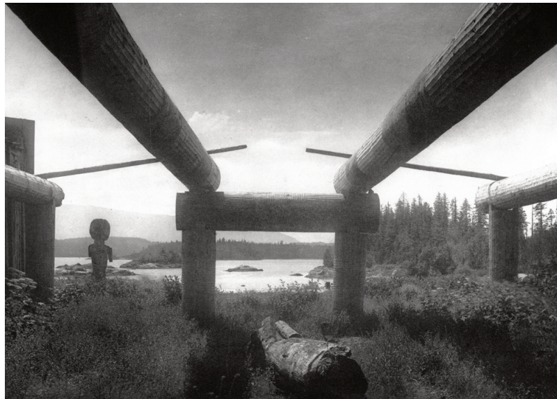
Figure 7.9 ▲ The framework of a large house with fluted beams in the Kwakiutl village of Mamalilikulla on Village Island, near Yalis (Alert Bay). Photo by E. Curtis. PN 2321, courtesy of the Royal BC Museum.
