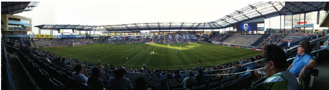
Figure 14.18 The Sporting Park in Kansas City, Kansas, is home to various sporting events. The stadium first opened for business in 2011, and taxpayers financed $146 million of the total cost to build the stadium, an office park, and a youth soccer complex. 85 (credit: Wesley Fryer)
