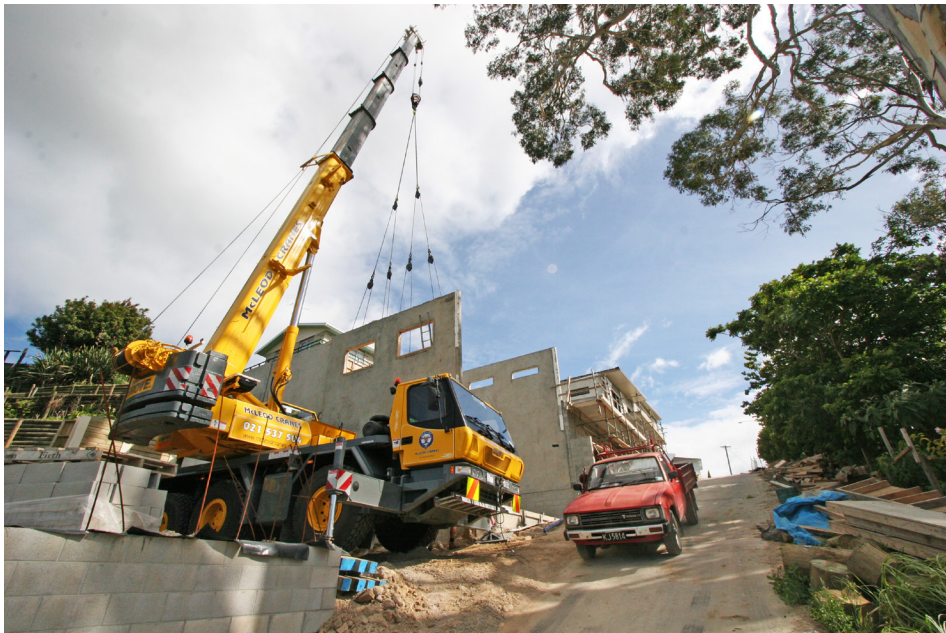
Figure 15 — Hydraulic boom truck crane
