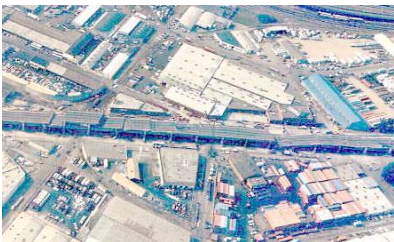
g / The collapsed section of the Nimitz Freeway.
