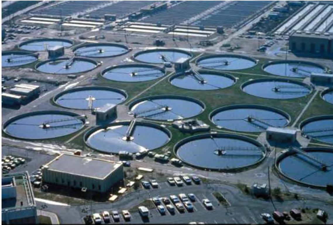
Figure 25.1 Sewage Treatment Plant (credit: "eutrophication&hypoxia"/flickr.com)
