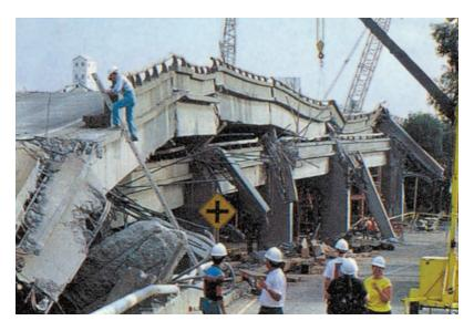
Figure 11.17 A part of the Cypress Freeway in Oakland California that collapsed during the 1989 Loma Prieta earthquake. [from: http://upload.wikimedia.org/wikipedia/commons/9/91/Cypress\_collapsed.jpg]
