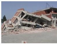
Figure 11.18 Buildings damaged by the 1999 earthquake in the Izmit area, Turkey. [from U.S. Geological Survey at: http://gallery.usgs.gov/sets/1999\_Izmit,\_Turkey\_Earthquake/thumb/\_/1]
