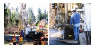
Figure 14.10 A water-well drilling rig in operation in the Cassidy area, near Nanaimo, B.C. In the photo on the right the well is being test-pumped with air pressure. The casing (yellow arrow) is about 40 cm in diameter. [SE]
