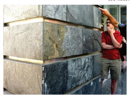
Figure 20.17 Slate used as a facing material on a concrete building column in Vancouver [SE]  $\,$
