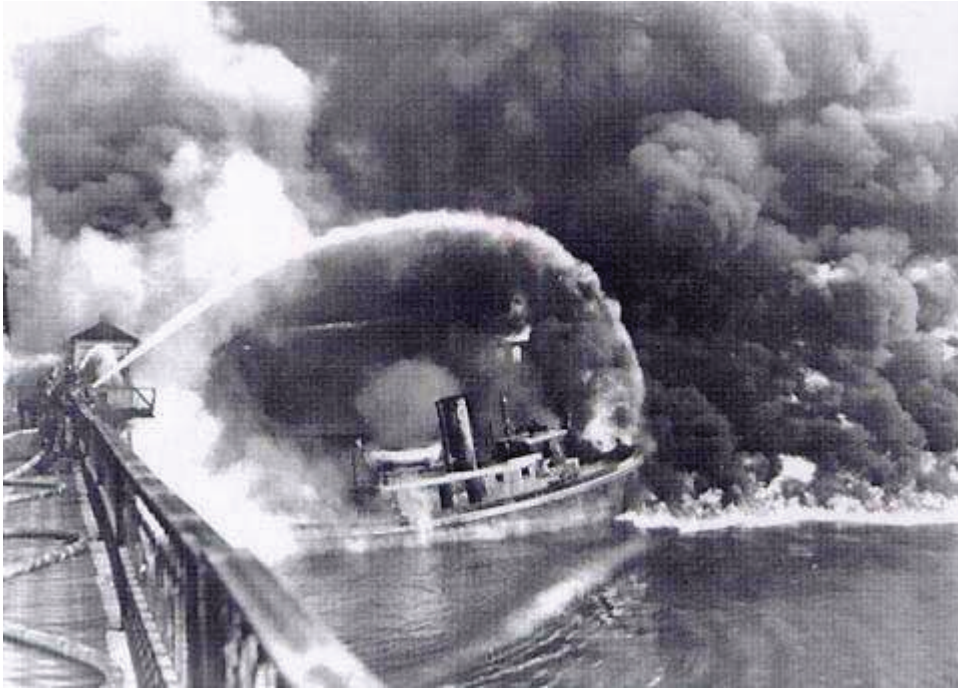
Figure 3. Cuyahoga River on fire. Source: National Oceanic and Atmospheric Administration
