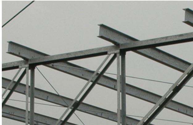
Figure 12.21 Steel I-beams are used in construction to reduce bending strains. (credit: modification of work by “US Army Corps of Engineers Europe District”/Flickr)
