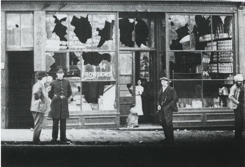
Building damaged during Vancouver riot of 1907 - 130 Powell Street. UBC Archives, JCPC_36_017.
