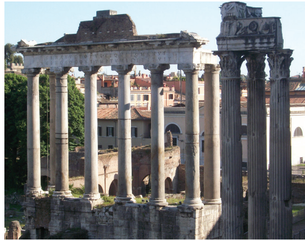
Figure 12.3 | This is a picture of the Roman Forum. Why did the Romans use so many vertical columns to hold up the one horizontal beam? If the horizontal beam spanned a long distance without support, it would buckle under its own weight. This beam is under tensional stress, so it is not as strong.
