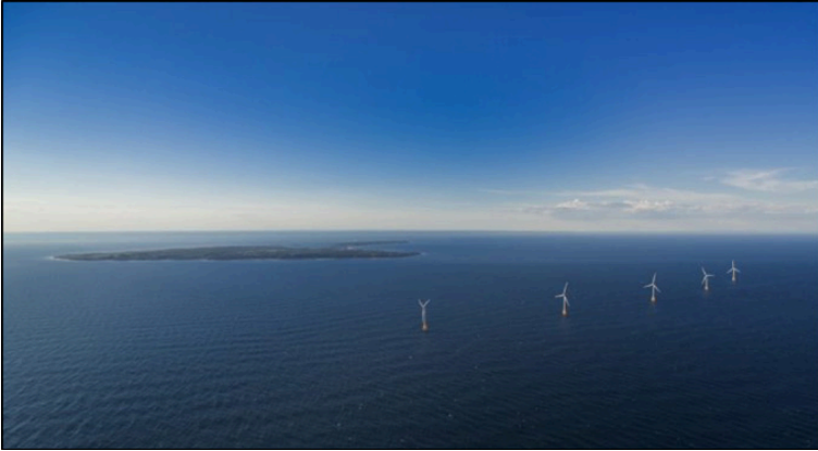
Figure 8.4: Block Island Wind Energy Installation, 2016 (Rhode Island)
