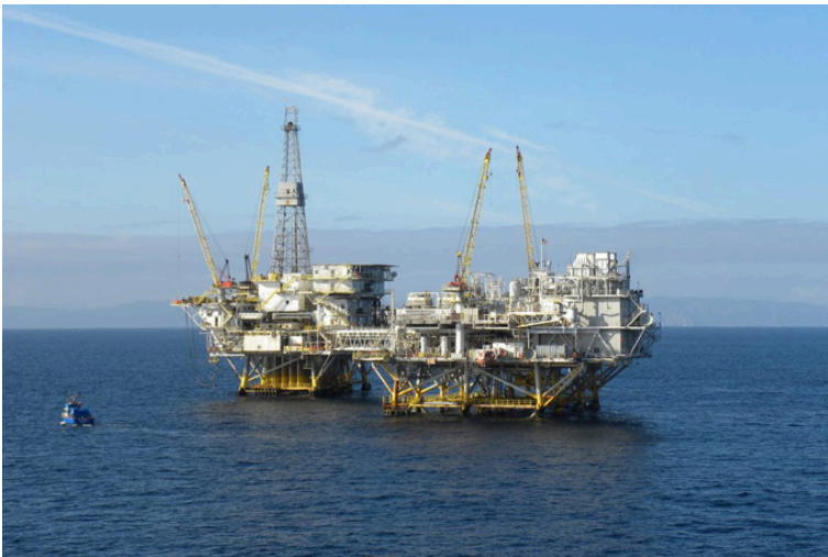
Figure 8.3 Offshore Oil Rig. From Bureau of Safety and Environmental Enforcement .
