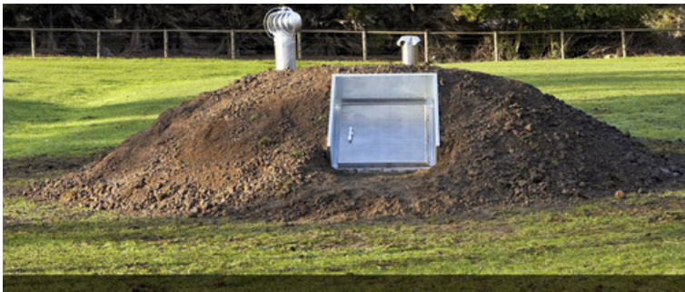
Photo 38: A Wildfire Safety Bunker
