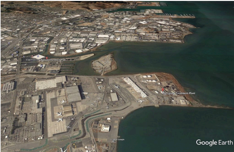
Figure 81: San Francisco and Mel Leong wastewater treatment plants, San Francisco Bay, California, USA
