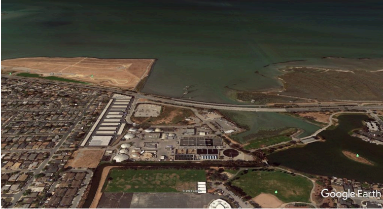
Figure 80: San Mateo wastewater treatment plant, San Francisco Bay, California, USA
