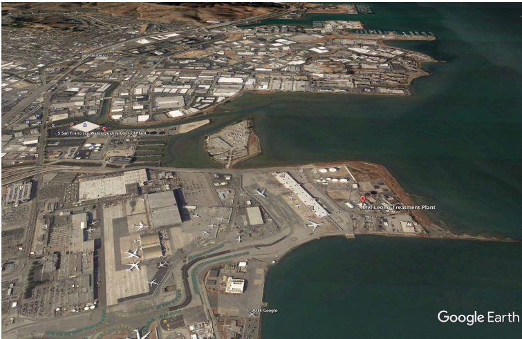
Figure 81: San Francisco and Mel Leong wastewater treatment plants, San Francisco Bay, California, USA
