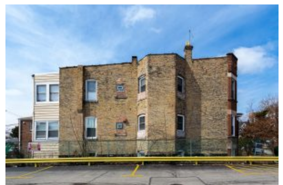
On buildings in Chicago, face brick is only a small sliver of brick facing the street, seen on right. Most of the rest of the building is made of Chicago common brick. Photo by Will Quam.
