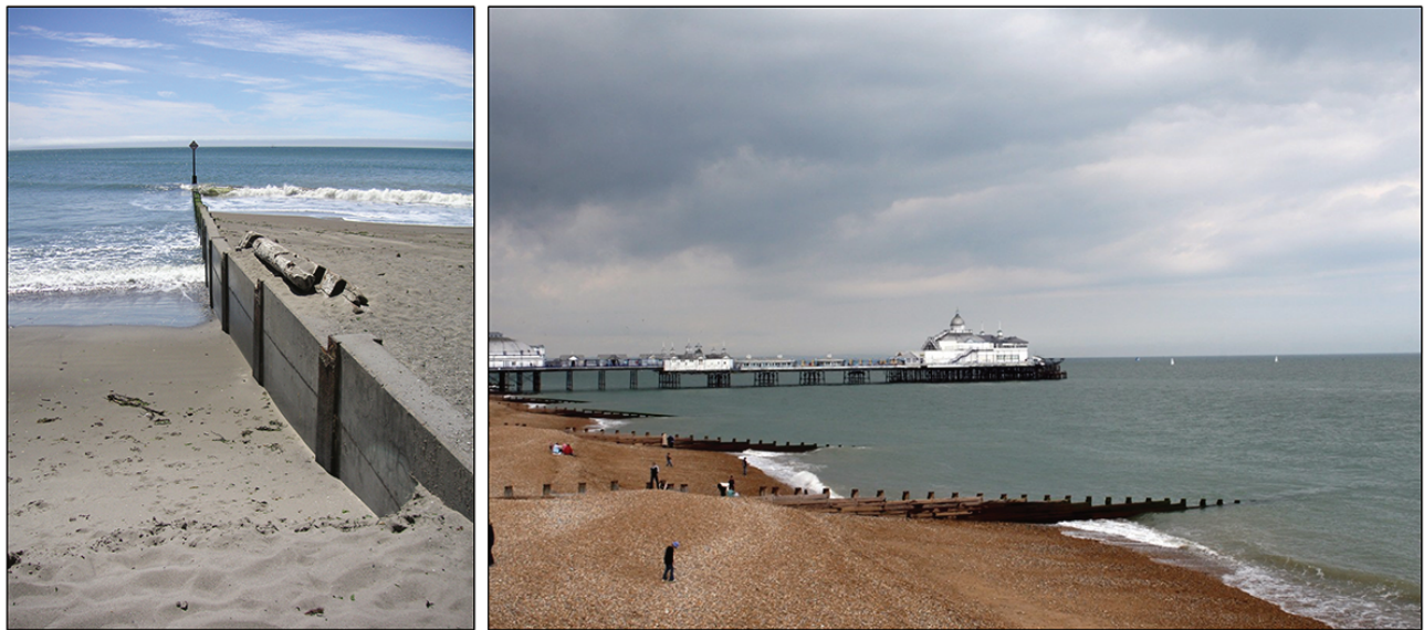
Figure 13.5.1 Left: A groin on Bolinas Beach, California. Longshore transport would be moving from right to left, accumulating sand on the right of the groin (Beatrice Murch, https://www.flickr.com/photos/blmurch/952523971 , CC BY-SA 2.0). Right: A groin field. Longshore transport would move from the bottom of the picture towards the top ( https://pxhere.com/en/photo/1048378 , Public Domain, CC0).
