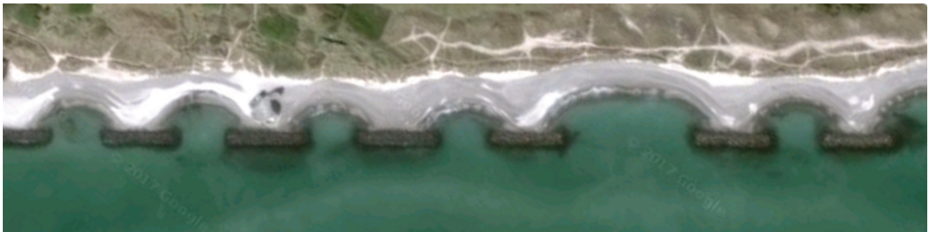
Figure 13.5.3 A series of breakwaters along the coast in Skagen, Denmark. In this case, sand has accumulated to the point that they now connect the breakwaters to land (Google Maps; Imagery: DigitalGlobe, Aerodata, International Surveys, TerraMetrics, Data SIO, NOAA, US Navy, NGA, GEBCO, Map Data: Google).
