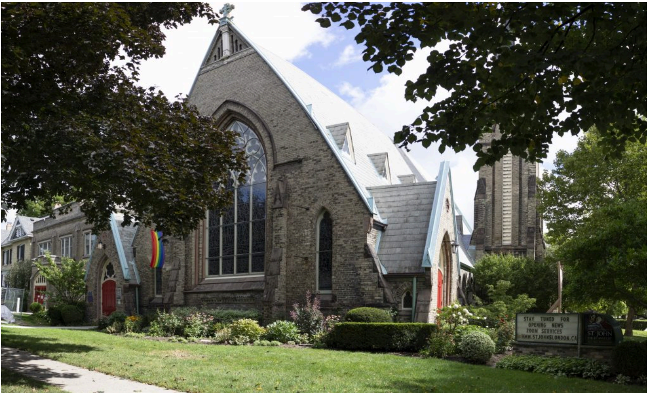
Church of St. John the Evangelist. View from the West. London, Ontario (Photograph: Anahí González).
